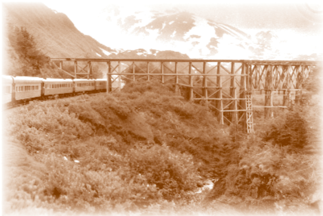
A train goes under the loop track where it crosses over itself during the summer of 1950. (ARRC photo archive)
