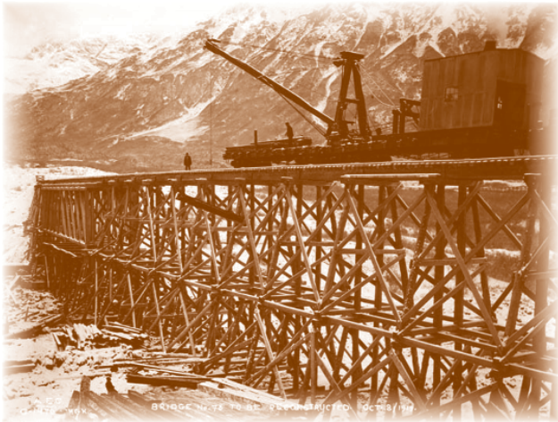
While some timber trestle bridges — such as the bridge at mile 75 that was reconstructed in 1919 — are tall and elaborate...
