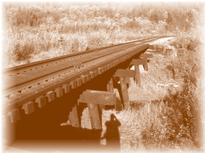
... Most timber trestle bridges are simple, utilitarian structures — such as this bridge at mile 335.8 (ARRC photo archive)
