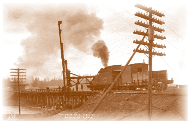
Alaska Engineering Commission crews employ a steam-driven pile driver to construct the bridge over Ship Creek. (ARRC photo archive)
