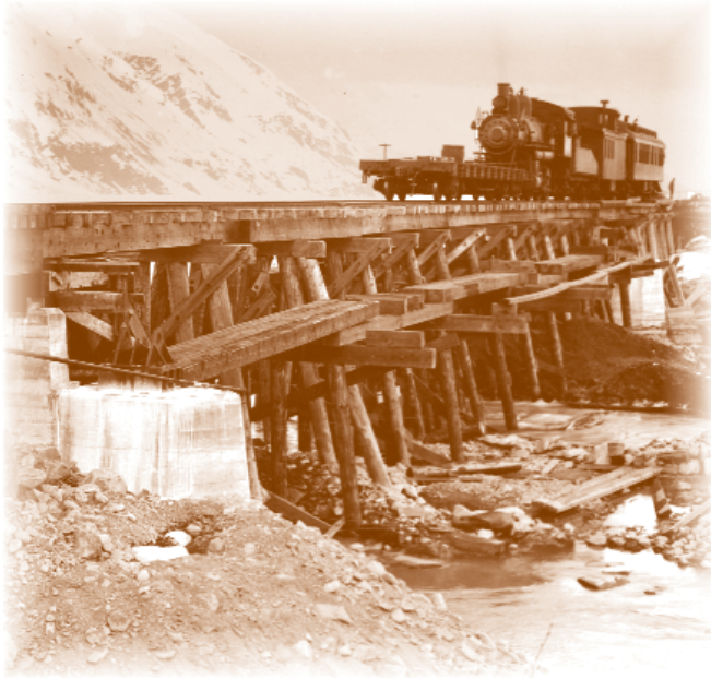
Bridge under construction at MP 54. (ARRC photo archive)
