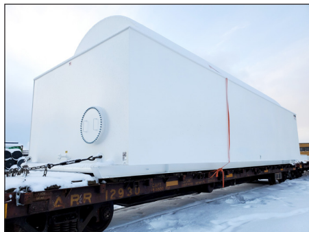
Modern 30,000-gallon fuel tanks are transported by rail and then lifted into place in January 2020
